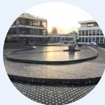
Permavoid subbase during installation
